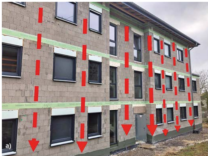
Fig. 12. Examples of favourable (a) and unfavourable (b) openings in external walls and the use of products with higher compressive strength in highly stressed areas
