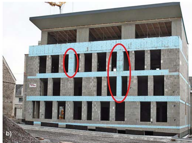
Fig. 12. Examples of favourable (a) and unfavourable (b) openings in external walls and the use of products with higher compressive strength in highly stressed areas
